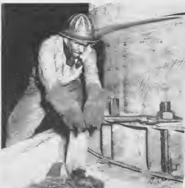
SNUGGING ANCHOR BOLTS that hold stack, is M. van der Linden. M. VAN DER LINDEN ta tene e staca na e base.
